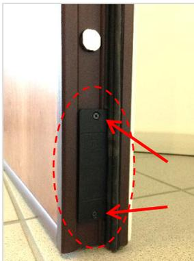
1. Find the battery pack position. This depends on door manufacturer. Usually it is installed in the front side of the door, up or down. In other cases, it can be placed in the top side of the door or even in the hinge side.
